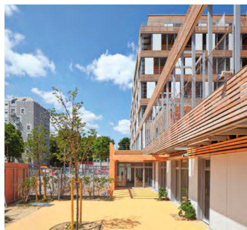
4 Rebière housing block Contracting authority: Paris Habitat – Project management: Belus
