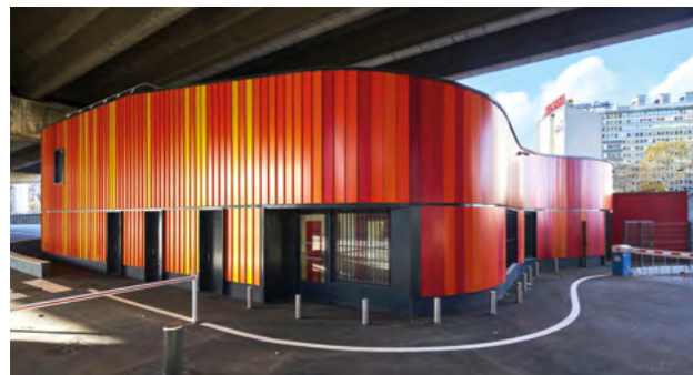
9 Car holding pond Project management: Gaia
