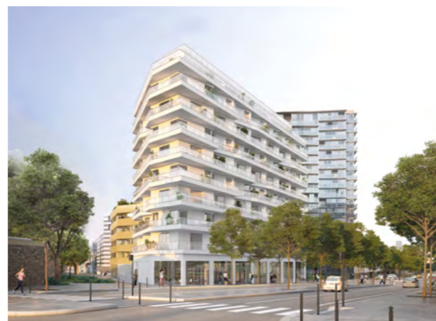
5 Social housing Project management: Lambert Lenack
