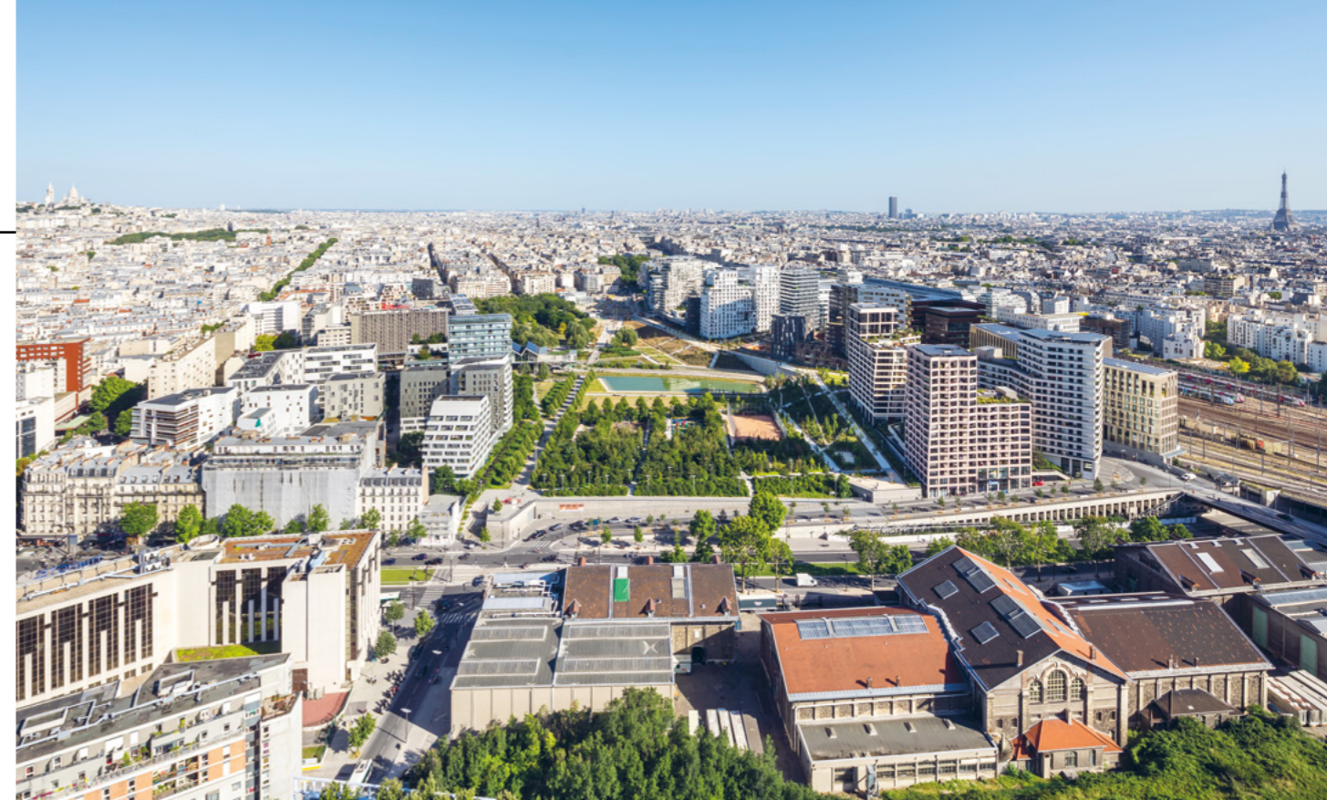
The West sector of Clichy-Batignolles is a major urban space (200,000 sqm of mixed-use developments) developed through collaborative design that combines multiple urban quality and usability objectives: wide-open landscape, new urban forms with buildings 50m high and complex high-density development with environmental goals.
