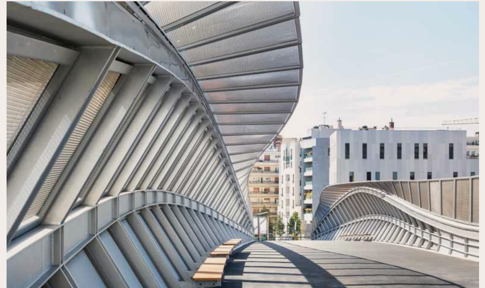
Passerelle Marcelle Henry, 2019 / Marcelle Henry footbridge, 2019
