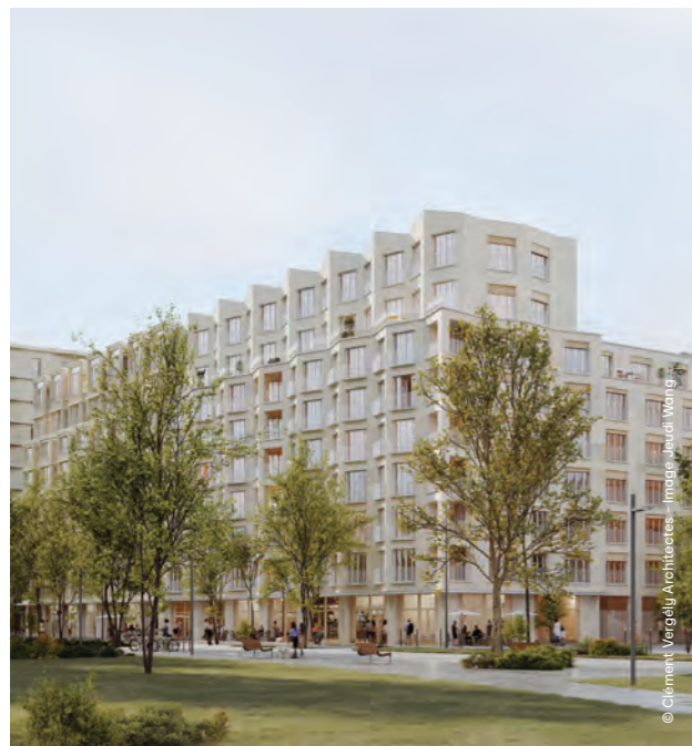
B2 Pitch Immobilier & Giboire: Clément Vergély architectes → 4,464 sqm of affordable housing for purchase (62 dwellings) → 241 sqm activities/shops Facade: self-supporting stone
