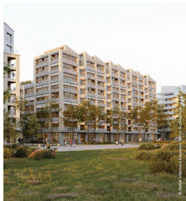
C RIVP: Atelier Villemard Associés + Heros Architecture → 6,234 sqm of housing (78 dwellings including 56 subsidised rented and 22 capped-rent) → 352 sqm activities/shops Facade: self-supporting stone
