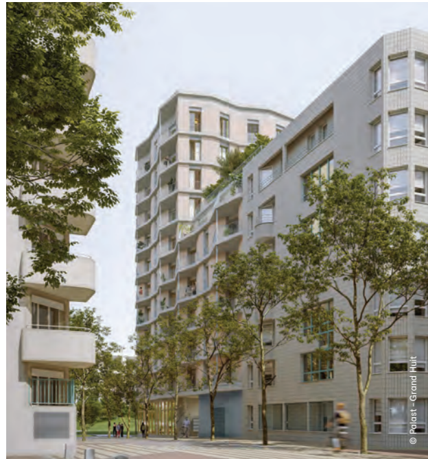
A RIVP for La Foncière de la Ville de Paris: Palast + GrandHuit → 2,386 sqm of housing under long-term lease scheme for low-income households → 126 sqm of activities/shops Facade: Wood frame facade with chopped straw + render
